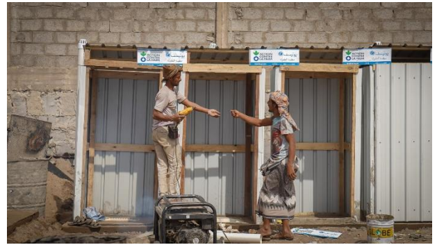
©UNICEF Yemen/2020. Construction of emergency latrines in Aden.
