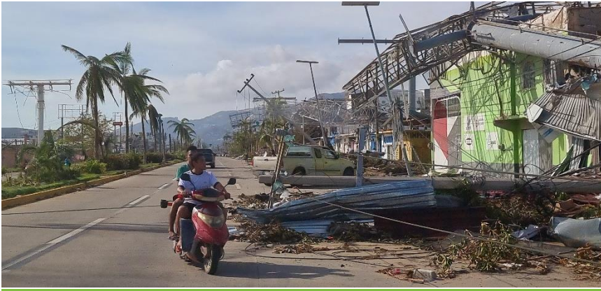
Photo: General view of damages in Punta Diamante – a touristic zone -, Acapulco, 3 days after the hurricane Otis made landfall. © UNICEF México/Andrés Ramírez Reporting period: 25 - 31 October 2023
