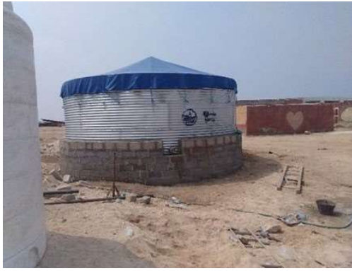
©UNICEF Yemen/2020 Installation of T-tanks for Kamran Island
