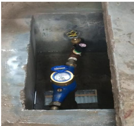
Picture 4: Metered water connection provided by DWASA
